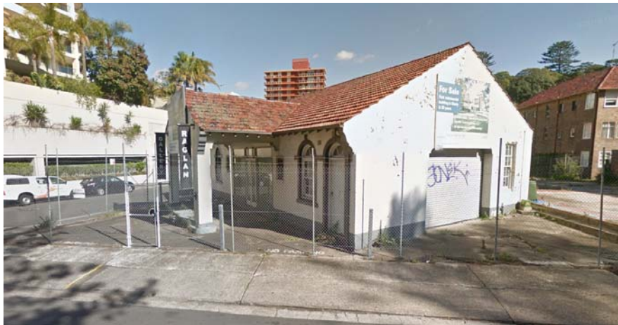
Existing Auckland Garage
